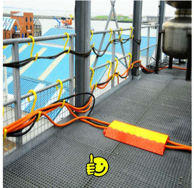
Using these Safety Hooks makes it extremely easy to suspend cables, electrical wires, hoses, and other work lines. They contribute to improved accessibility by clearing the work floor, and greatly reducing tripping hazards. First introduced in Europe in 1994, these hooks have been used successfully in many plant construction, turnaround, and maintenance situations.
