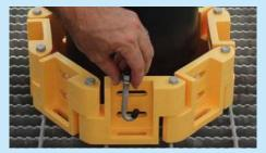
Drop J-bolts in the slots located on the bottom of each T5-J piece. Catch one of the grating bars with the J-bolt and tighten. Do this for all T5-J pieces.
